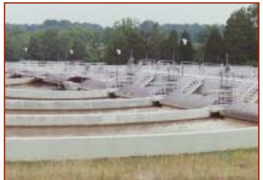
MSD's regional wastewater treatment facilities are recognized by the Association of Metropolitan Sewerage Agencies for performance excellence.
