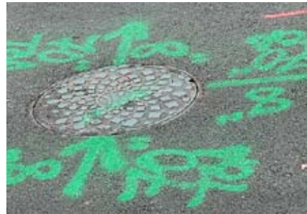
BUD markings indicate the location of underground utility facilities.
