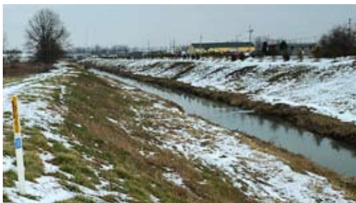
The Northern Ditch Interceptor will be constructed along the channel beginning east of National Turnpike and continuing to Outer Loop.
