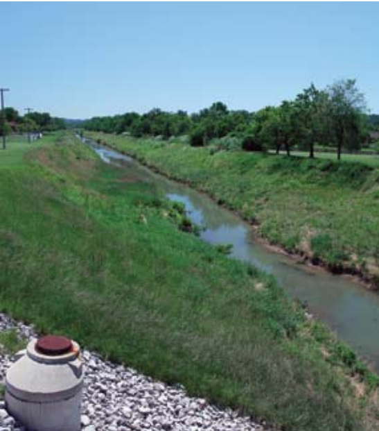
The Northern Ditch Interceptor will carry wet weather flow from the Highgate Springs area to the Pond Creek Interceptor to prevent pumped sanitary sewer overflows during rain events.
