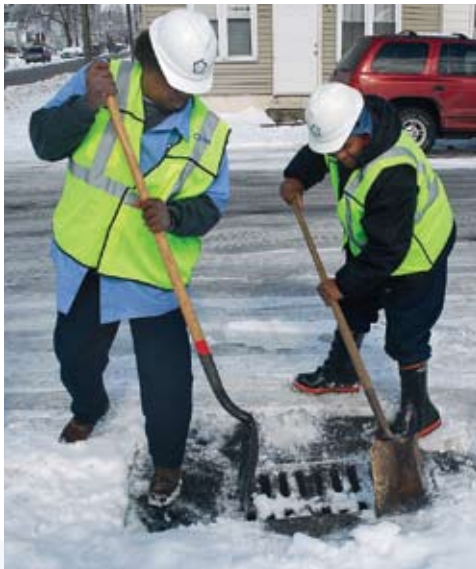
Butch O'Bannon (left) and Keith Brooks cleared snow and ice from a drainage inlet to prevent water ponding on the roadway.
