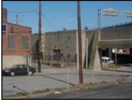
Figure 19. 10th St. Flood Pumping Station
